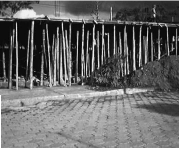
Figure 4. Use of bamboo poles for support in traditional construction.
