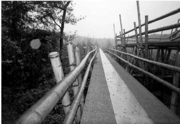
Figure 1. Bamboo bridge in the Amsterdamse Bos (photo by Pablo van der Lugt).
