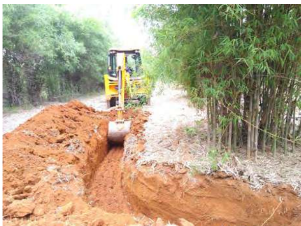
Fig 2. Spiral trenching using JCB in D. stocksii plantation
