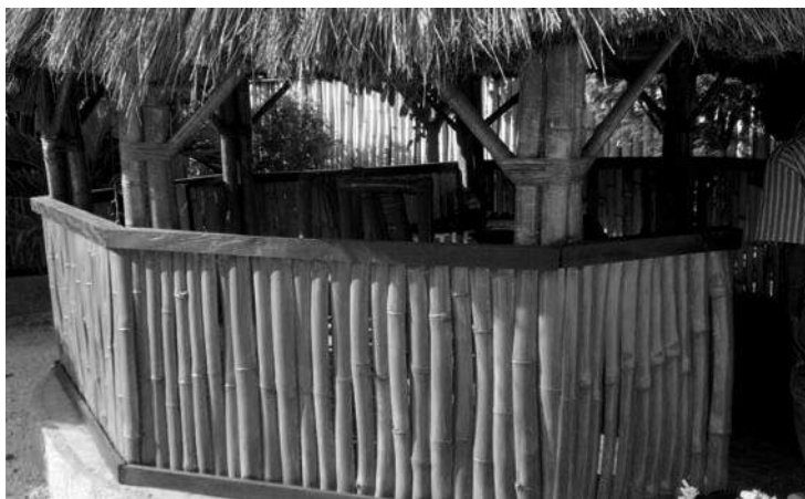
Figure 2: Use of bamboo in 'summer hut' construction at Cape Coast, Ghana
